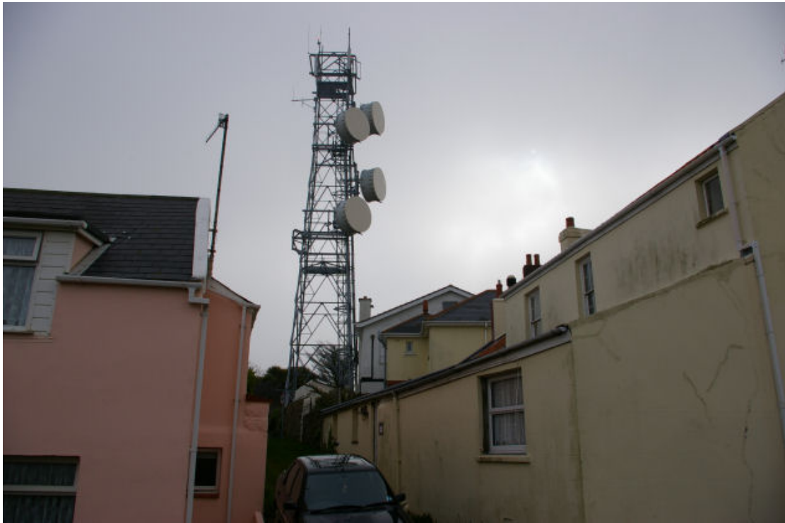
Figure 3 – The mast at Alderney Exchange
