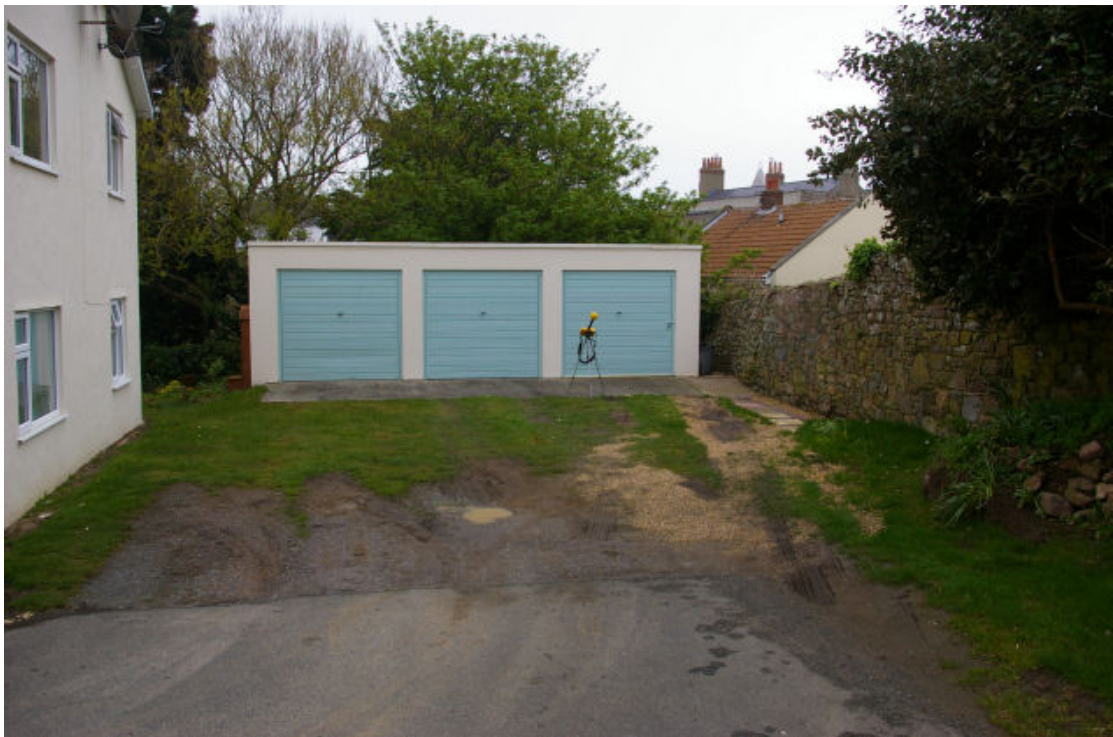
Figure 4 – EM Probe at Alderney water tower – Loc 1 (All Peaks)
