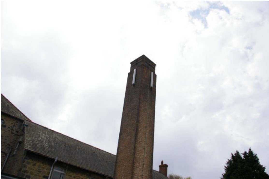
Figure 3 – The antennas at the site in Castel Hospital are attached to the chimney
