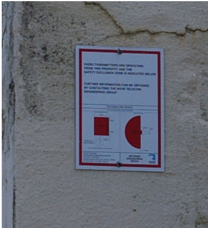
Figure 5 – Hazard sign posted on the wall next to the antenna. The sign describes the extent of the exclusion zone
