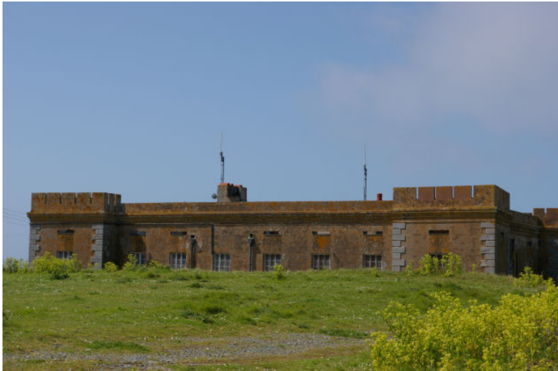
Figure 3 – Antennas at the Fort Richmond site
