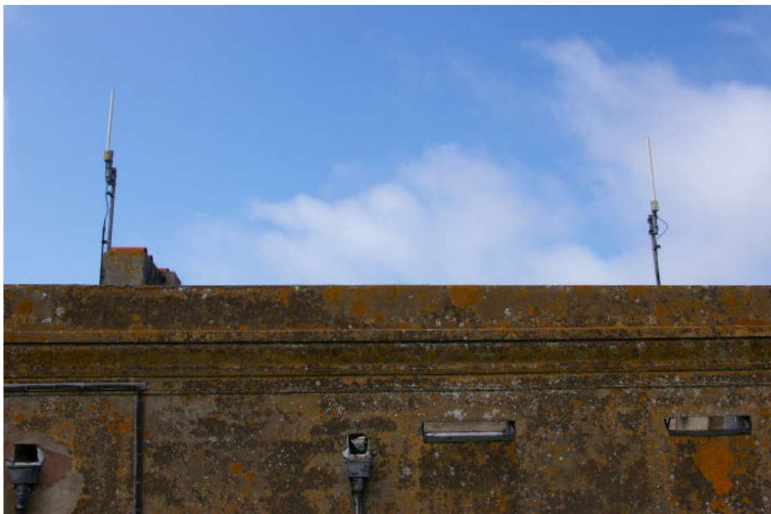
Figure 4 – Detail of the rooftop antenna installation
