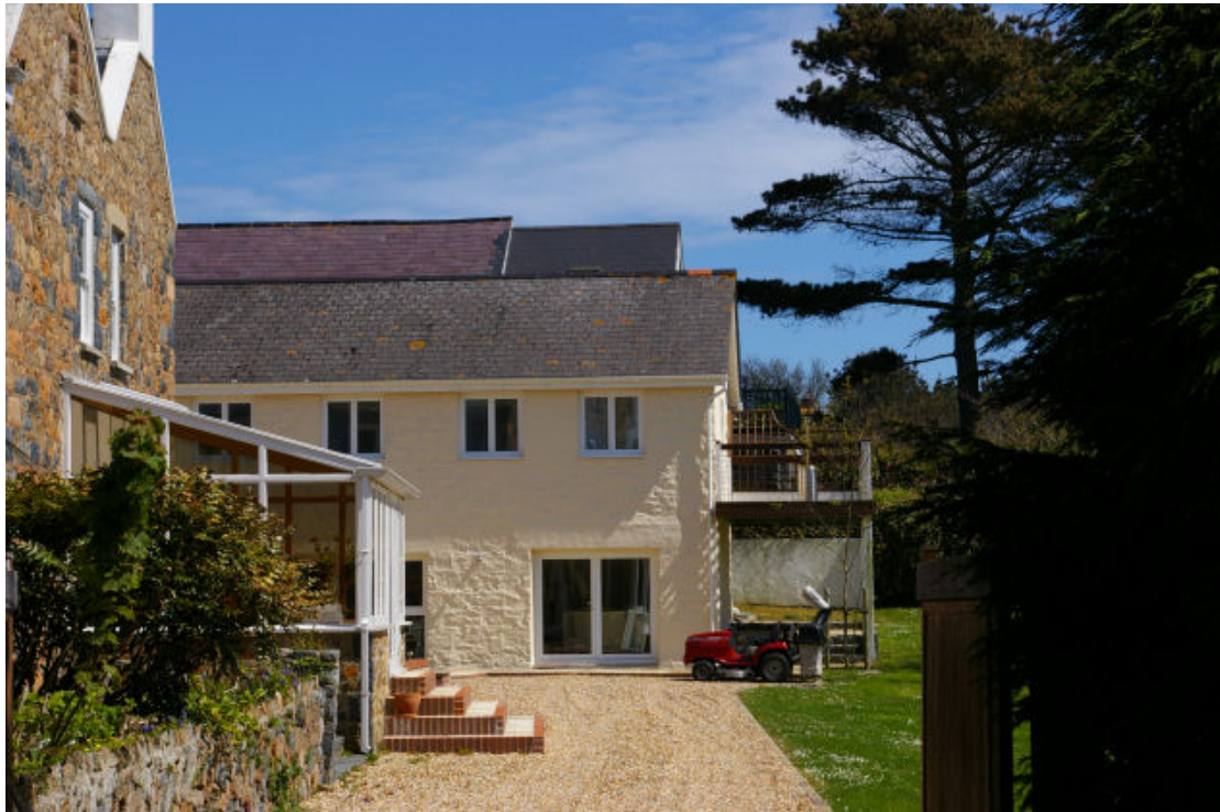
Figure 3 – The site antenna at Gouffre are located within the loft space of a private residence
