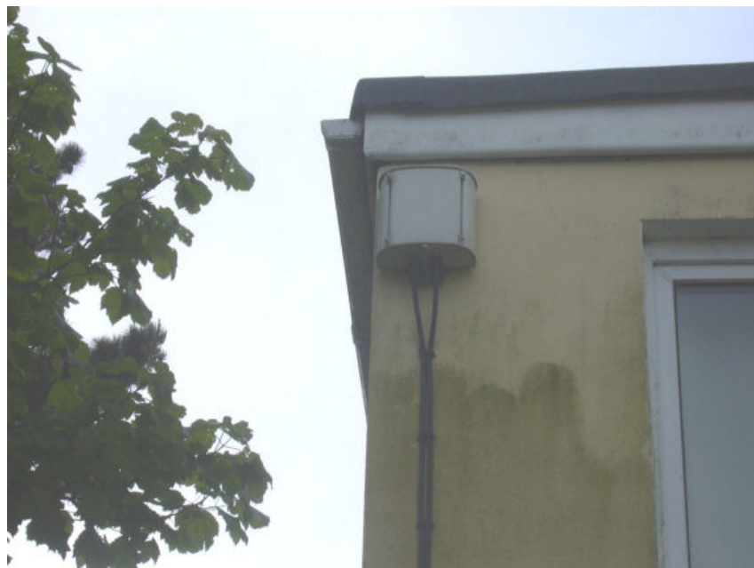
Figure 4 – Detail of the antenna installation
