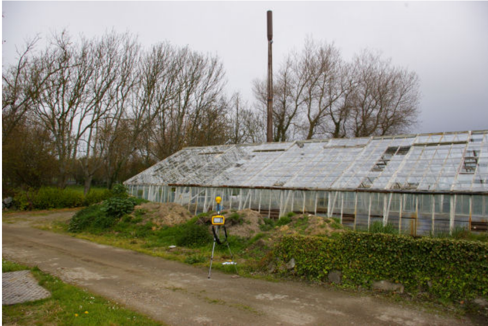
Figure 3 – Probe location at Marais Vinery, with the existing mast in the background
