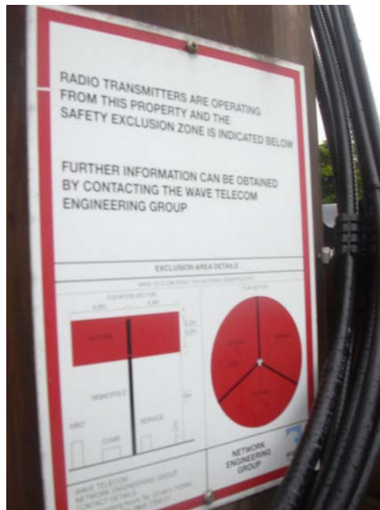
Figure 4 – RF hazard sign posted at the foot of the mast showing extent of the exclusion zone
