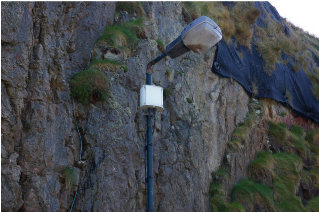
Figure 4 – Antenna Installation (Detail)
