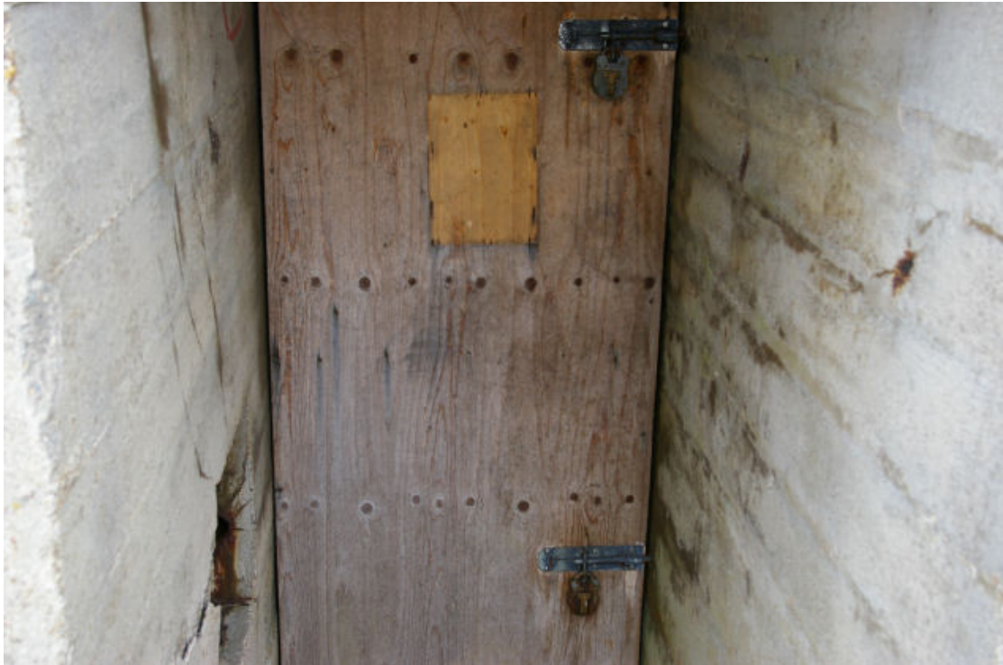
Figure 5 – Access to the rooftop is restricted
