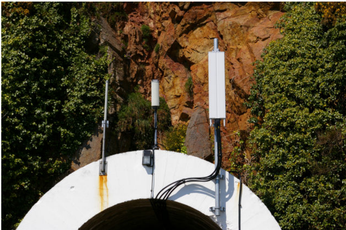
Figure 4 – Antenna Installation (Detail)
