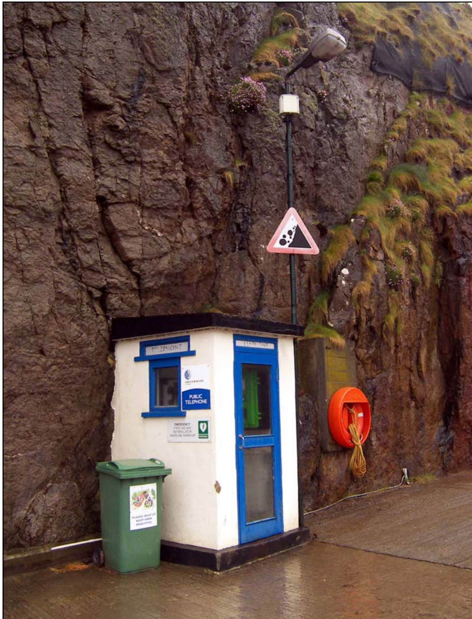
Figure 3 – View of the External Antenna (attached near top of lamp post)
