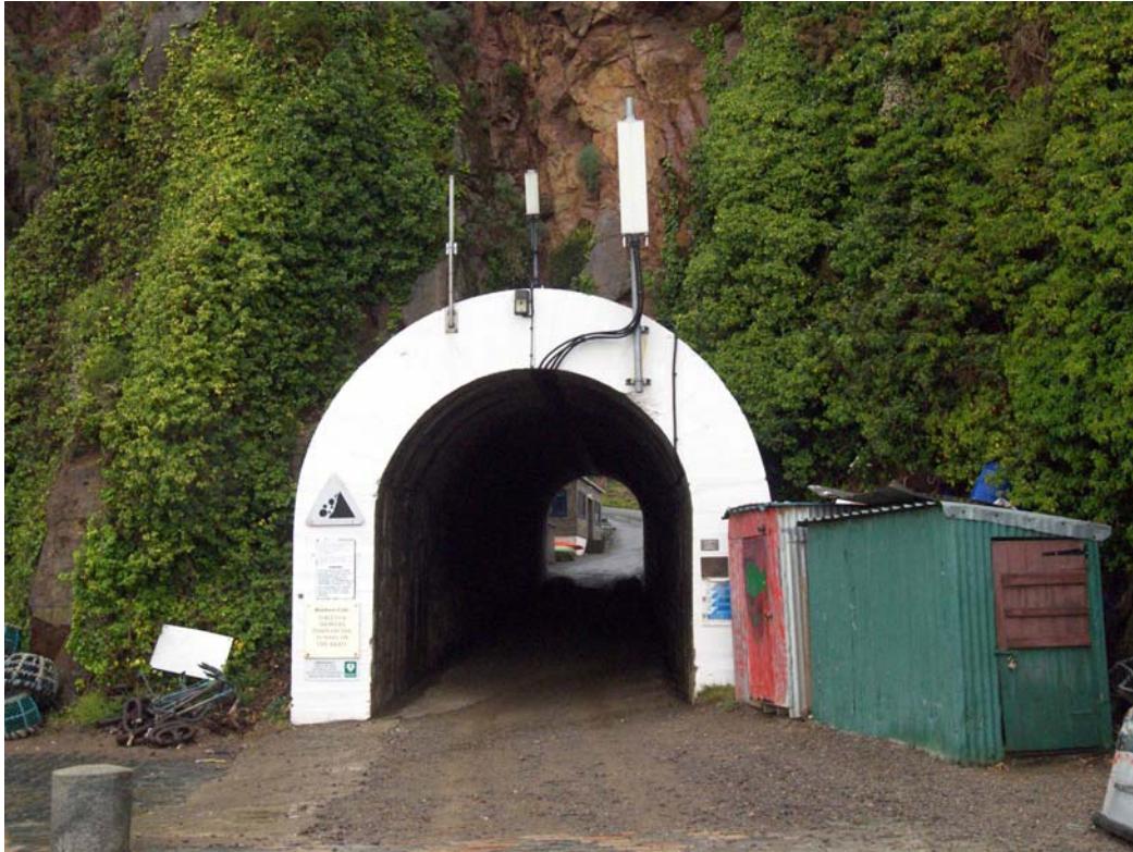
Figure 3 –View of the three antennas at the entrance of the tunnel
